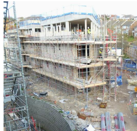
East block under construction
