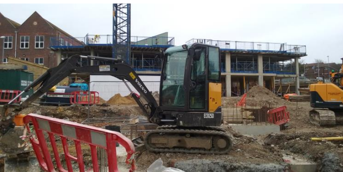
Work underway at Hobby Place
